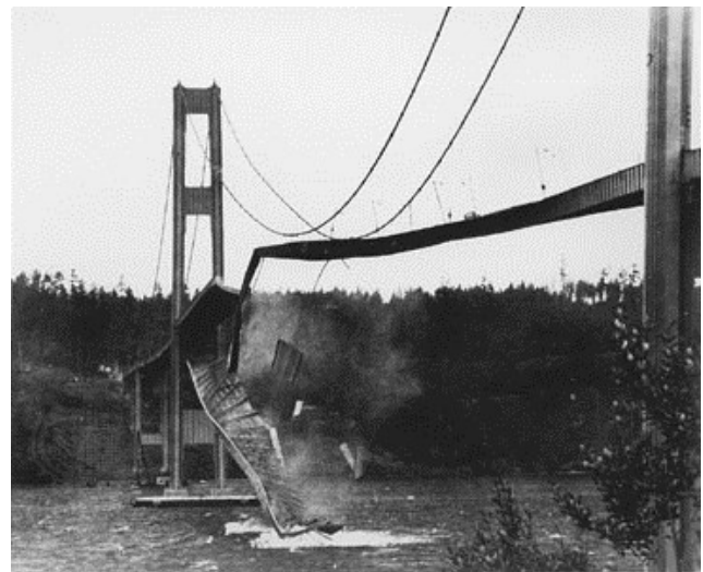
Tacoma Narrows Bridge collapse [8]
